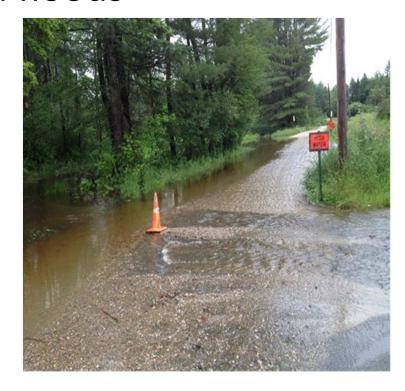
• The Town has applied for a Hazard Mitigation grant to replace the two existing 48" culverts with a 4'x8' box culvert similar to the one under Route 4.
