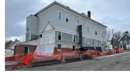
What are helical piles and what do they do? Helical piles provide foundation support. This is particularly important if the soils are not ideal. Many years ago, following a fire at this location, the remains of the building were pushed behind Whitney Hall and paved over. These organic materials are less stable as they are still decomposing. Helical piles are screwed into the earth. By embedding helical piles under the surface, the needed stability is provided for the building foundation.
