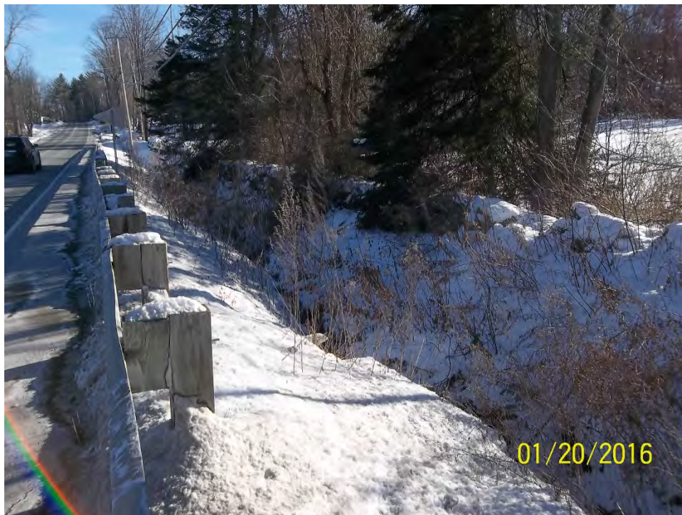
Photograph C8: Inlet drainage into culvert shown in Photograph C7. This area picks up drainage from subdivision development on Warren Road to right.
