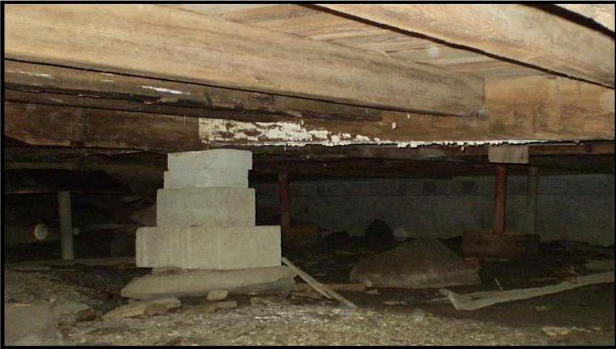
Figure 3 - Mold on girder. Note variation in/improvised nature of foundation support for floor system.
