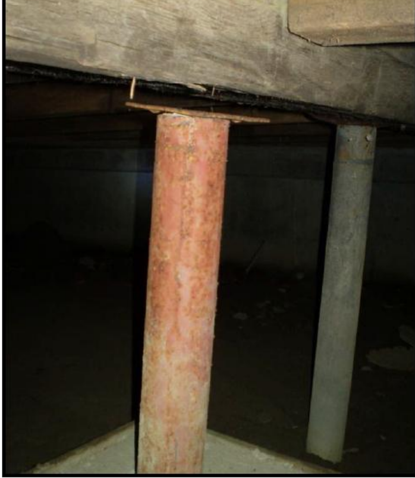
Figure 4 - Structural support post no longer in contact with underside of girder due to foundation settling.
