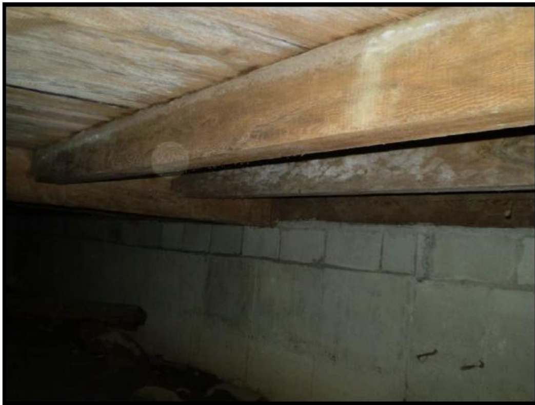
Figure 2 - Mold on joists and wood decking.
