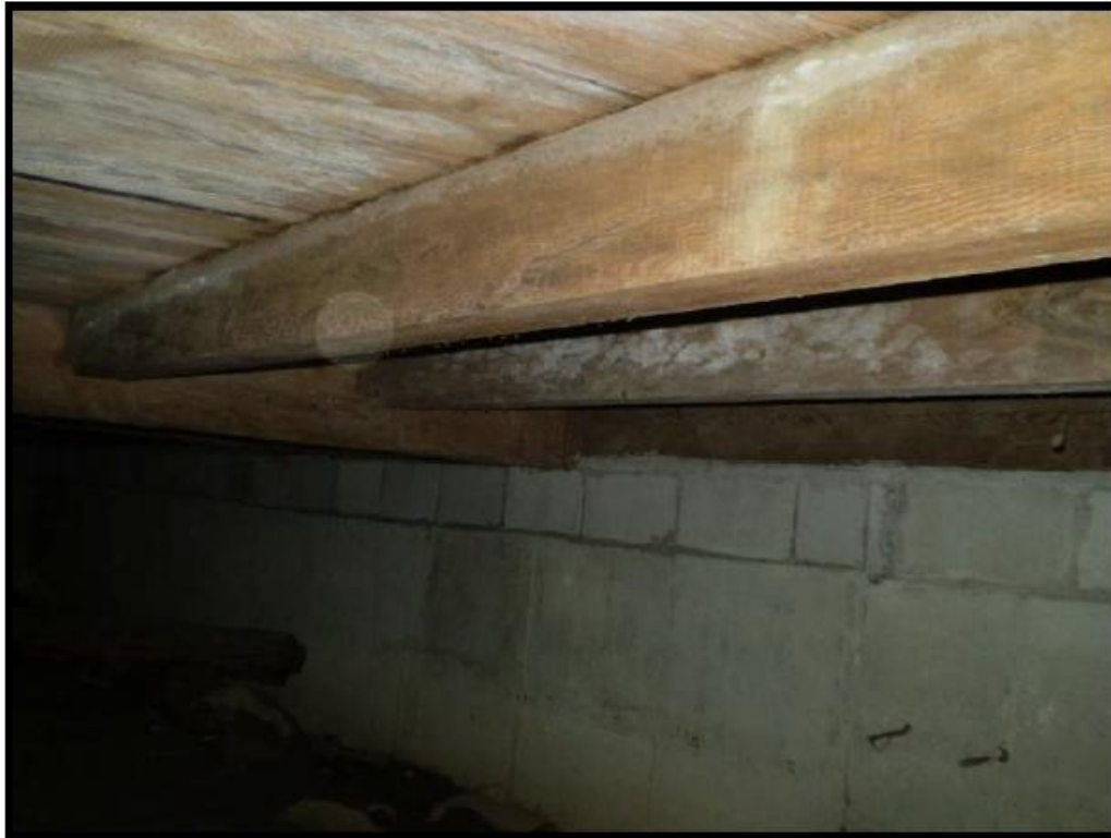
Figure 2 - Mold on joists and wood decking.
