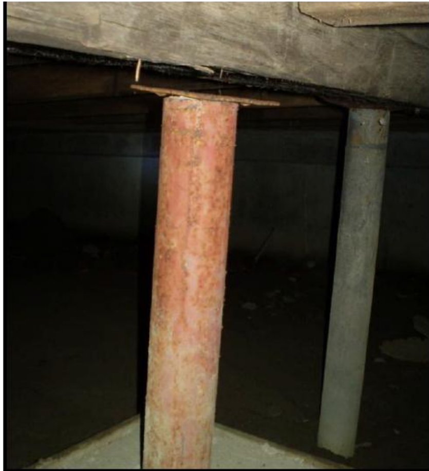
Figure 4 - Structural support post no longer in contact with underside of girder due to foundation settling.
