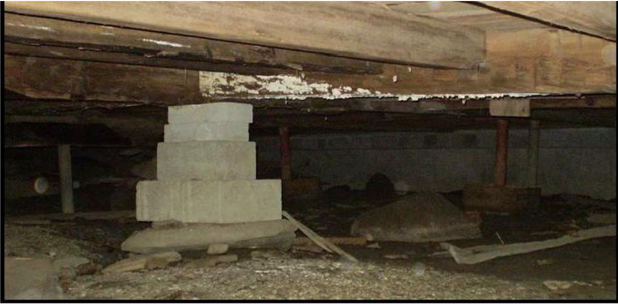
Figure 3 - Mold on girder. Note variation in/improvised nature of foundation support for floor system.
