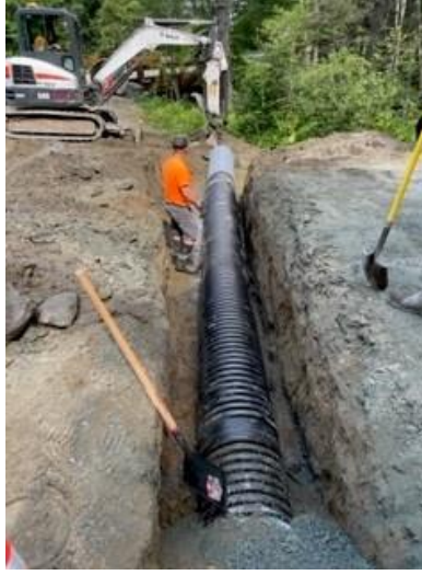
Figure 2 New Plastic Culvert being Installed.
