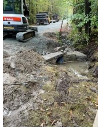
Figure 3 New Stone Headwall installed to protect pipe inlet.
