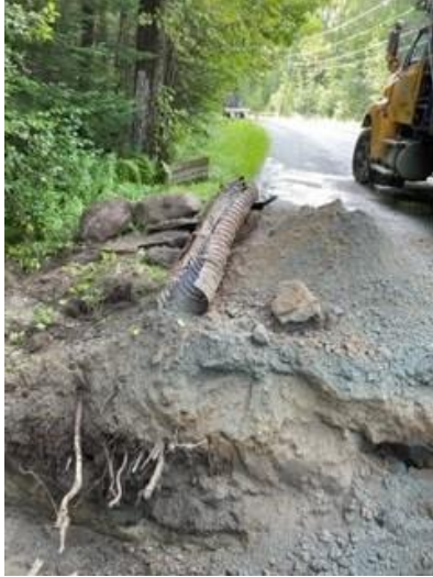
Figure 1 Failed Metal Culvert removed.
