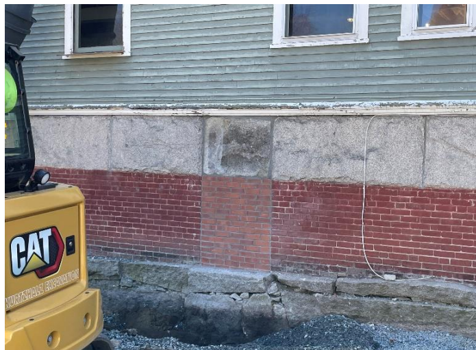
Window that had to be removed has been sealed up
