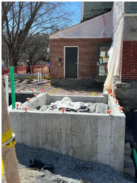
Foundation walls for new entrance before floor was poured
