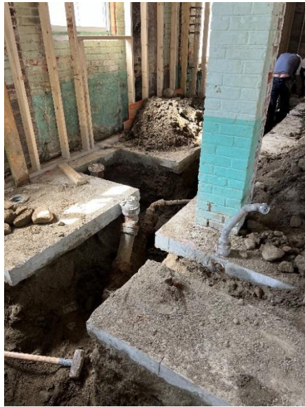
Trenches for new plumbing on ground floor
