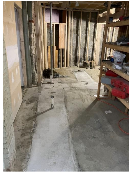
Trenches for new plumbing have been filled
