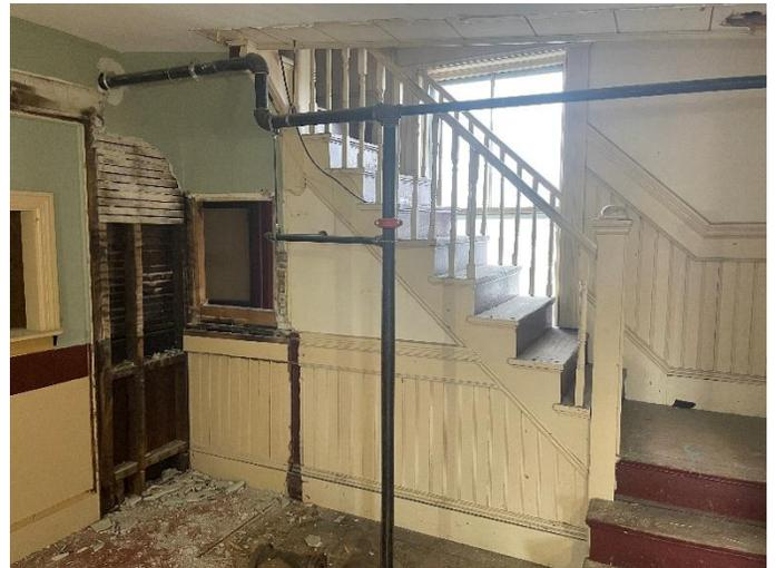
Interior work also continues with library restrooms removed and the wall and door at the bottom of the balcony stairs also removed.
