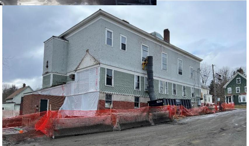
Work on the Whitney Hall renovation and expansion project continues. In February, the old vault was removed. As a cost saving measure, the elevator shaft and mechanical room will remain in their current locations. Foundation work for the addition also began. Helical piles are being installed to provide a stable foundation for the new structure.
