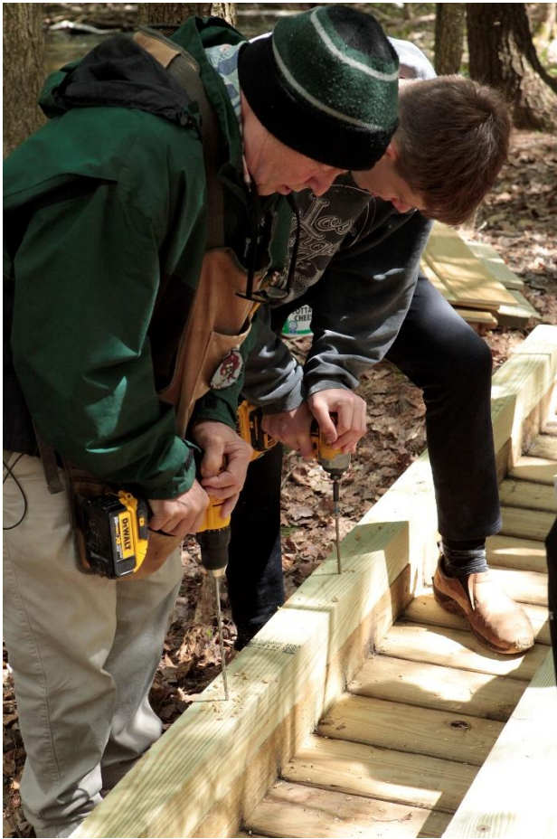
Installing timber screws to attach the double 4 x 4s together.
