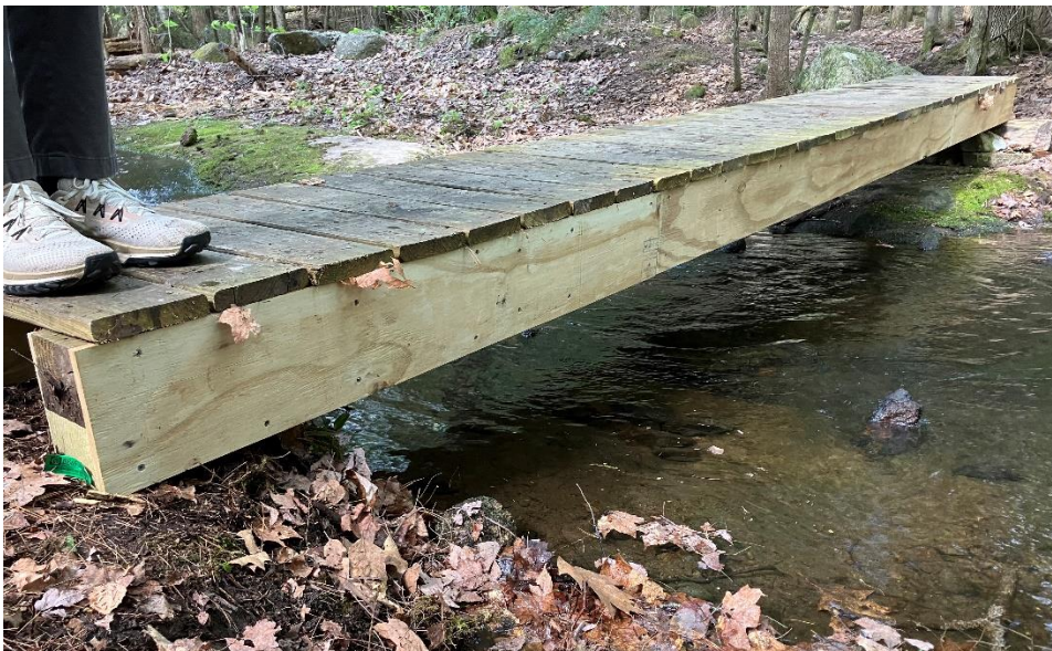
Plywood "gussets" were installed on either side of the double 4 x 4s to splint them together
