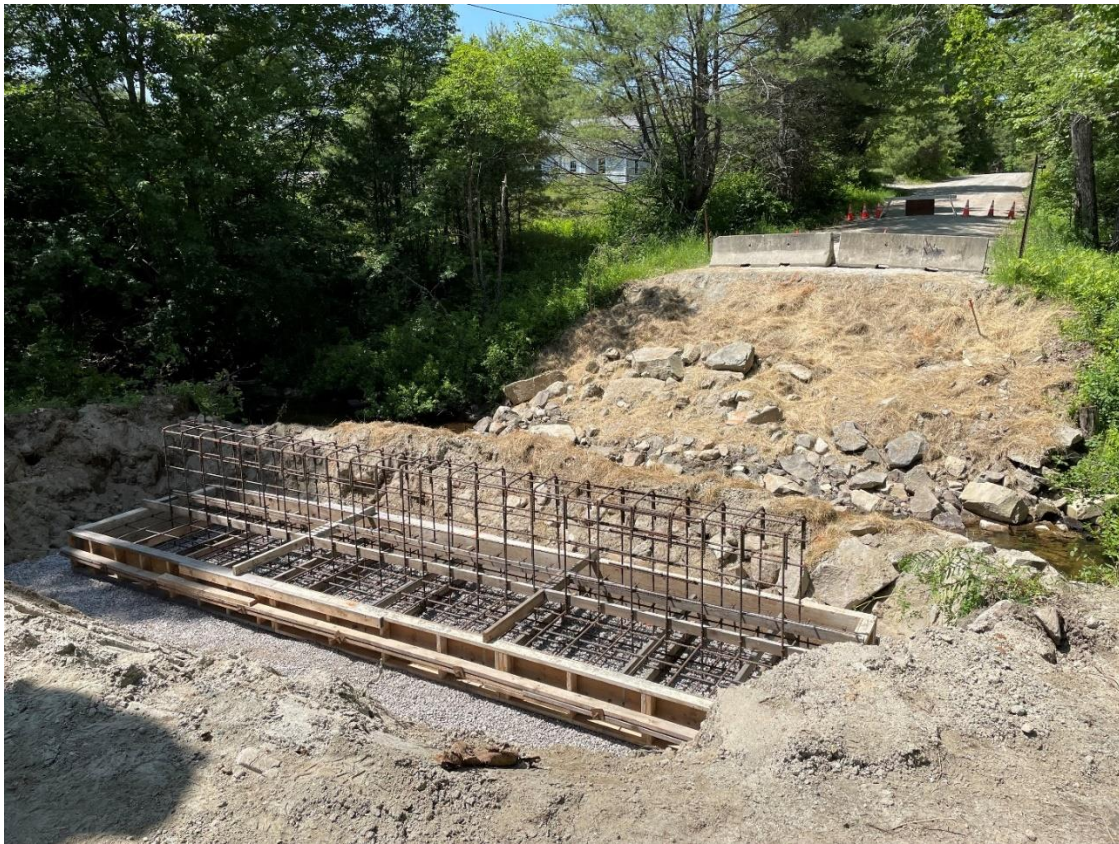
Photo: Oak Hill Road Bridge South Side Footing Ready for Concrete
